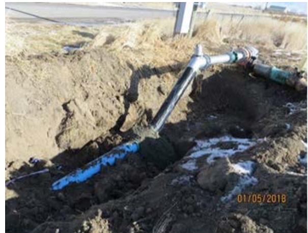
Sand Ridge Pipeline Installation
