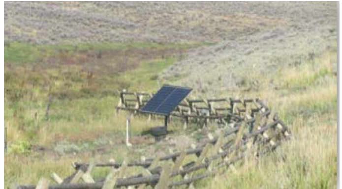
A pump powered by this solar panel operates a stock watering system in Humphrey
