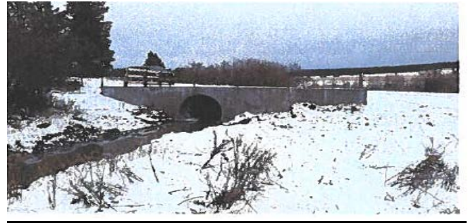
Keuterville Road Replacements
