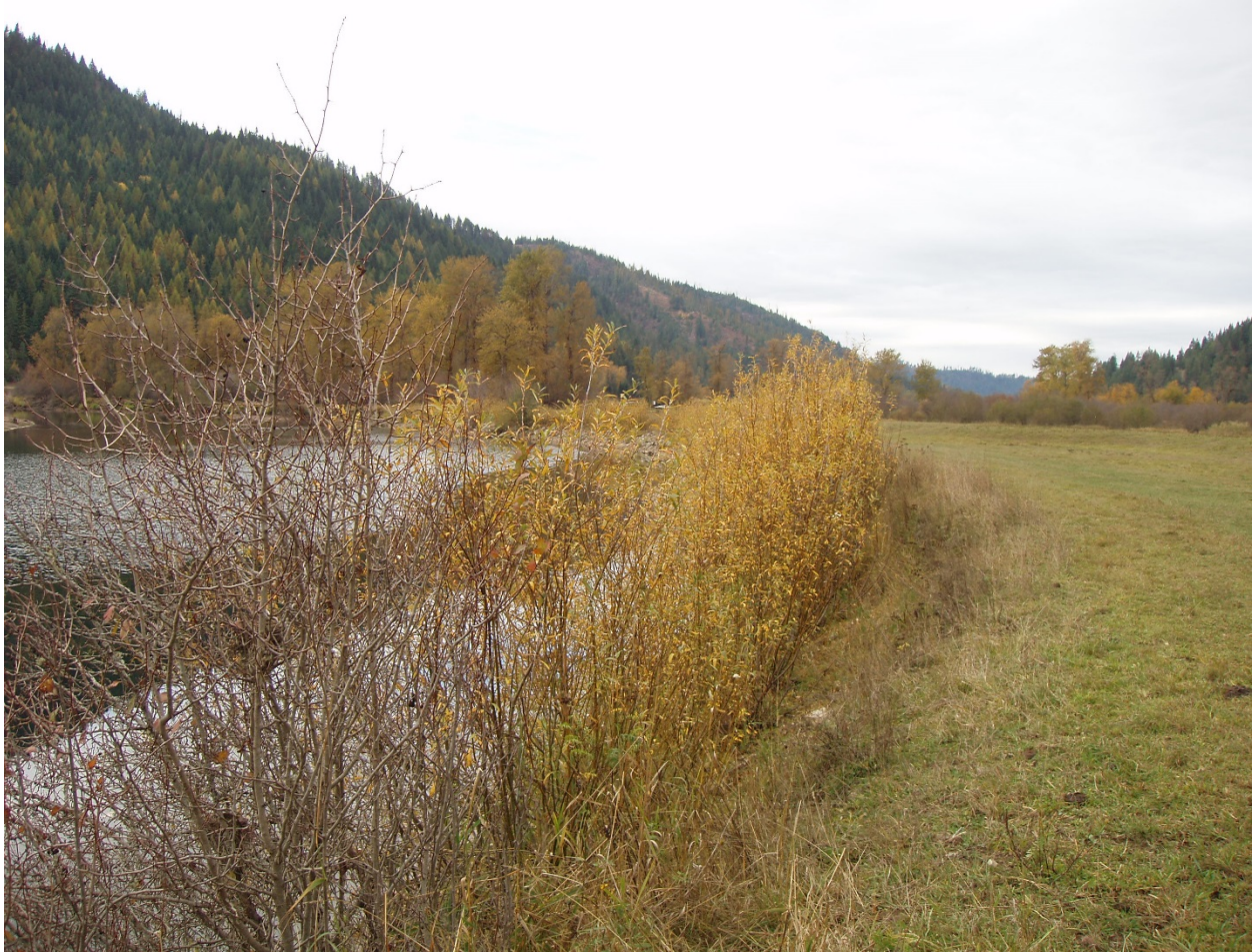
Figure 1: St. Joe River Streambank Protection with Rock and Vegetation
