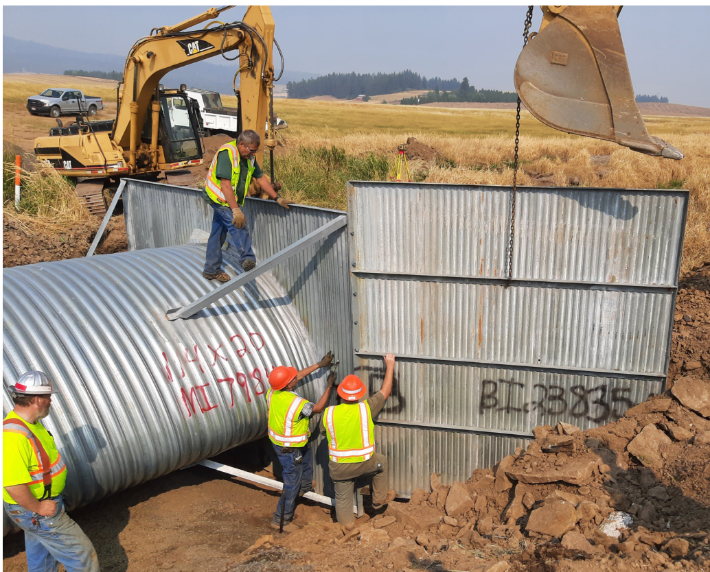
Clearwater Road Department employees install new Louse Creek culvert. Below, the new culvert in place. (photo courtesy Clearwater SWCD)
