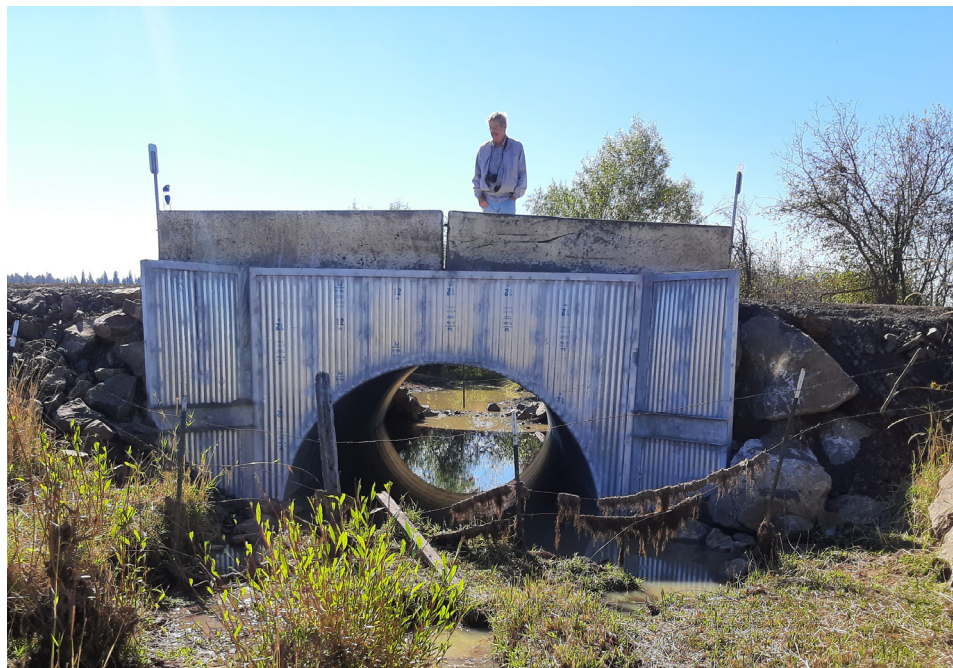
New Heywood Creek culvert installed (above). Old undersized culverts are shown below. (photos courtesy Clearwater SWCD)
