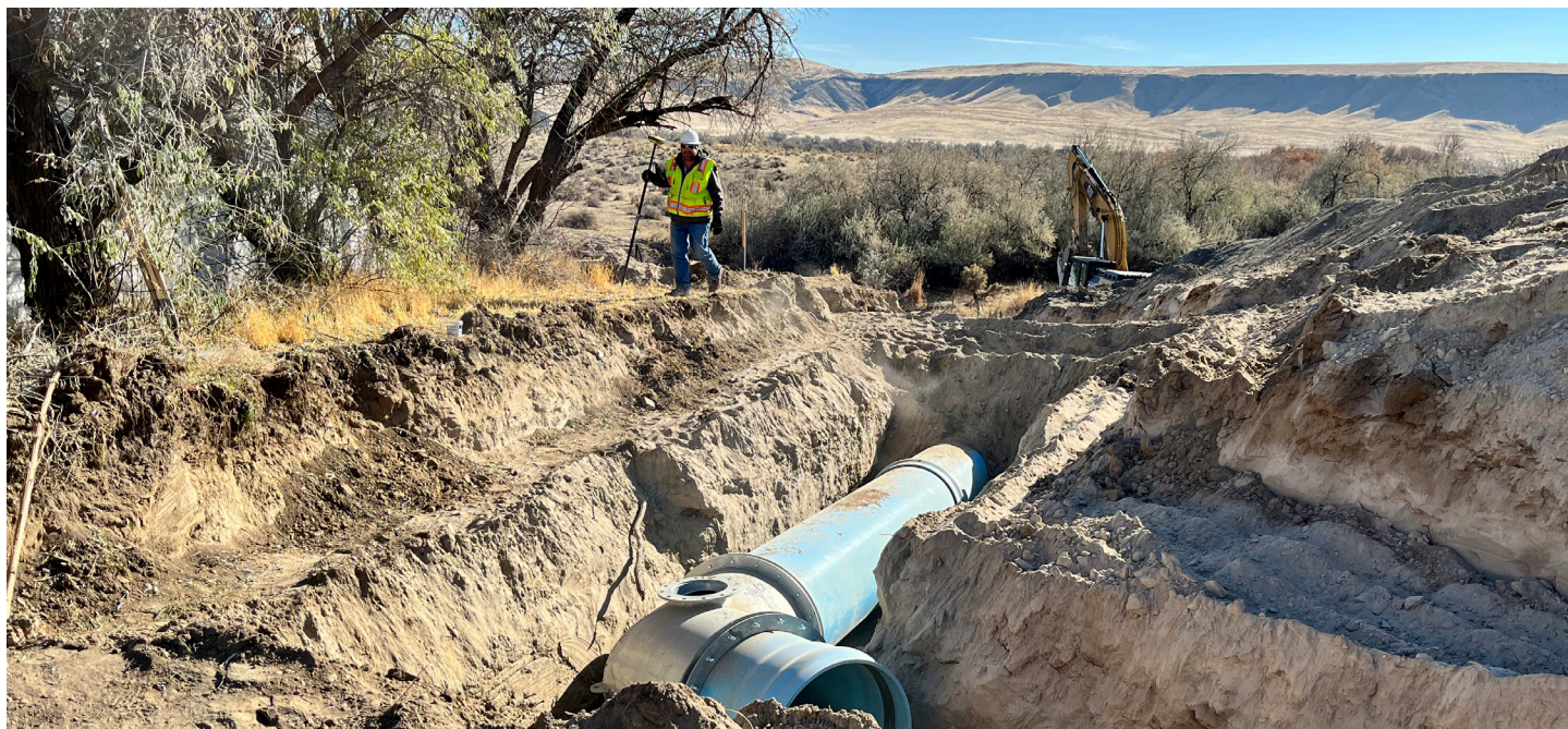
Contractors bury irrigation pipe just uphill from the Snake River near Hammett. (photo by Steve Stuebner)
