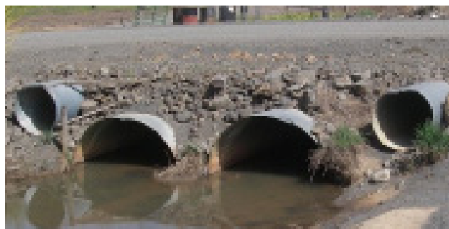
New Heywood Creek culvert installed (above). Old undersized culverts are shown below. (photos courtesy Clearwater SWCD)
