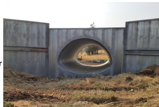
Clearwater Road Department employees install new Louse Creek culvert. Below, the new culvert in place. (photo courtesy Clearwater SWCD)
