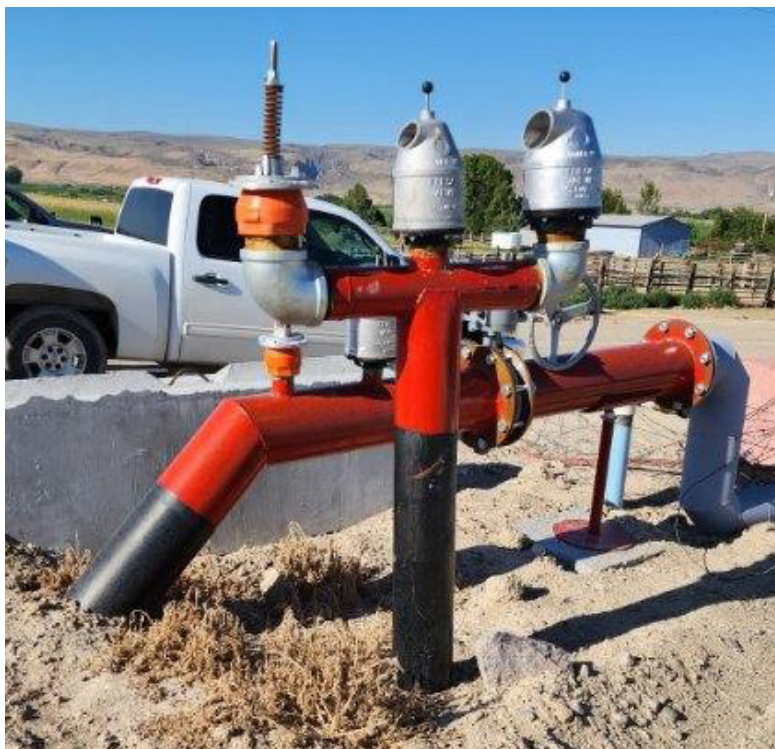
Left, Oteco pivot track filler in action. Right, pressurized irrigation system on the 26.9 Lateral canal provides a turnout at farm fields with pressure-relief valves and air vents to protect the new pipeline (courtesy Owyhee District).
