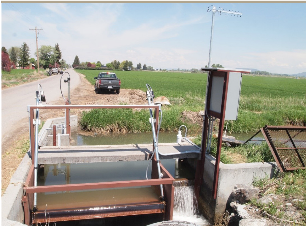
New automated headgates on the South Branch of the Parks and Lewisville canal system, funded by a WQPA grant via the Jefferson SWCD. (photo courtesy Jefferson SWCD)
