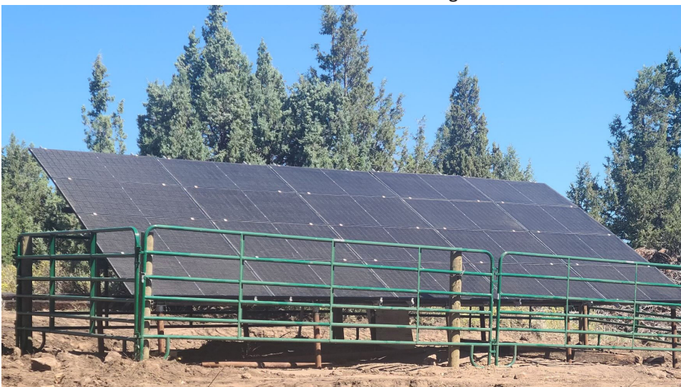
Marsh Valley ranchers installed a 8,000-watt solar booster system for pumping water uphill to off-stream cattle troughs with a USDA rural development grant.
