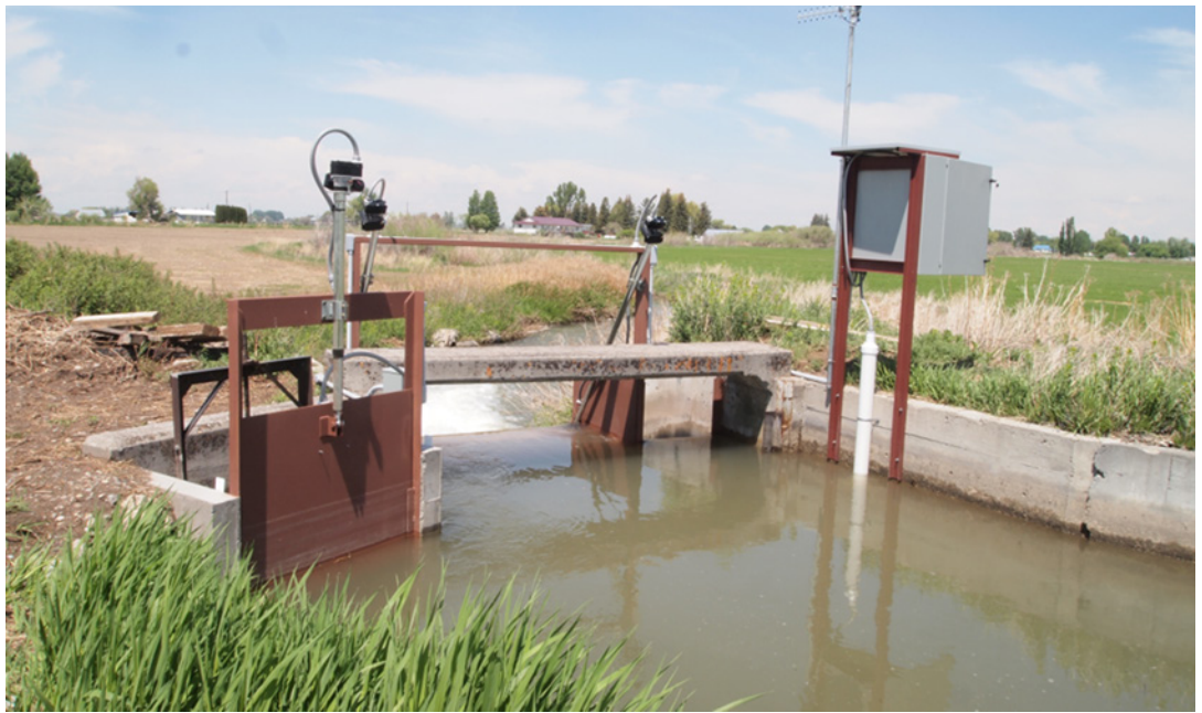
A WQPA grant funded three new headgates with automation for the Parks and Lewisville Irrigation Co. via the Jefferson SWCD. This is the Missionary Branch of the canal system. (courtesy Jefferson SWCD).
