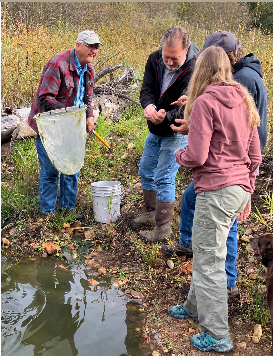
L-R, Steve Funk, SWC Engineer Bill Lillibridge, Paul Schelpp (contractor), and Jenna Ditzel with SWC, look at juvenile cutthroat trout that Funk wanted to save from the construction work. (courtesy Kootenai-Shoshone SWCD)
