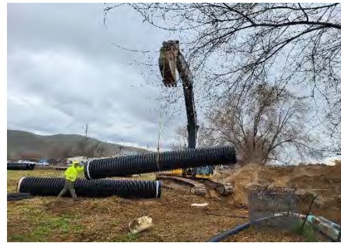
WQPA Underground Drain Replacement
