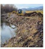
The Squaw Creek Streambank Improvement Project treated 3 sites of eroding streambank on Squaw Creek in Ola, Idaho, for a total of 460ft of improved streambank and 530ft of riparian fencing installed. This project decreased sediment load by 51 tons per year, nitrogen by 163lbs per year, and phosphorus by 82lbs per year.
