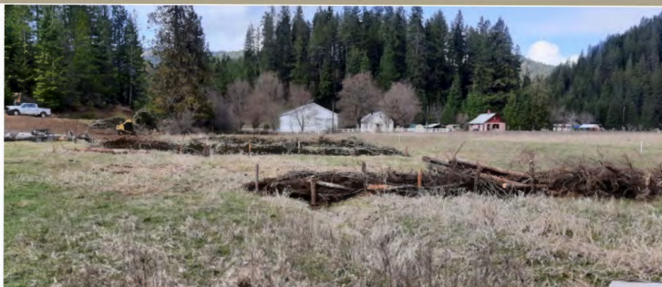
Above, two more PALS installed along Schlagel Slough. (photo by KSSWCD)
