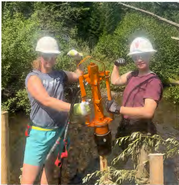
It’s hard work to run the hydraulic post-pounder but these two volunteers were up to the task! (photo by PCEI volunteers)
