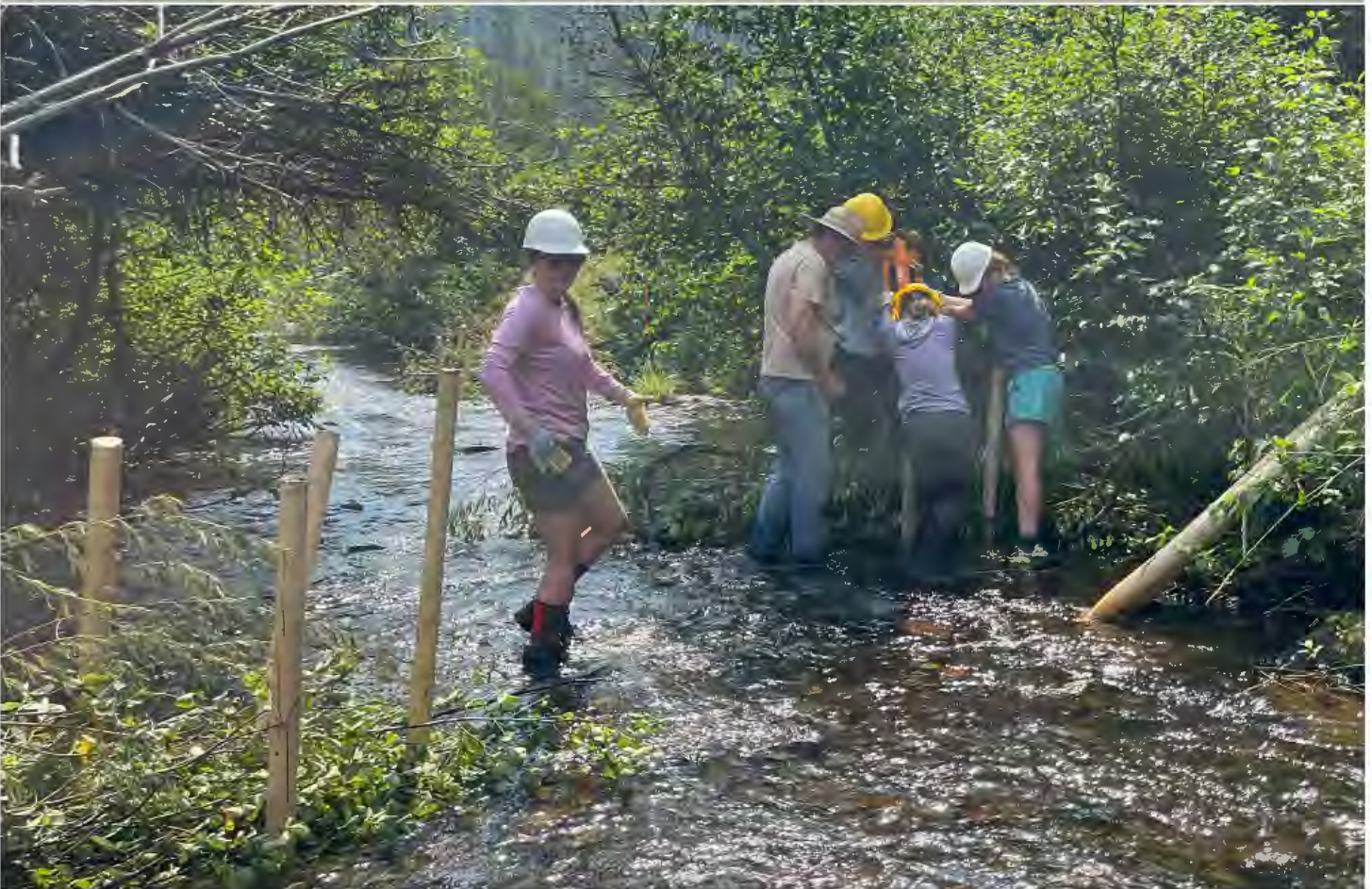
Volunteers install two Post-Assisted Log Structures (PALS) on the East Fork of the Potlatch River last summer. (photo by project volunteers, who were provided by the Palouse-Clearwater Environmental Institute and AmeriCorps.)
