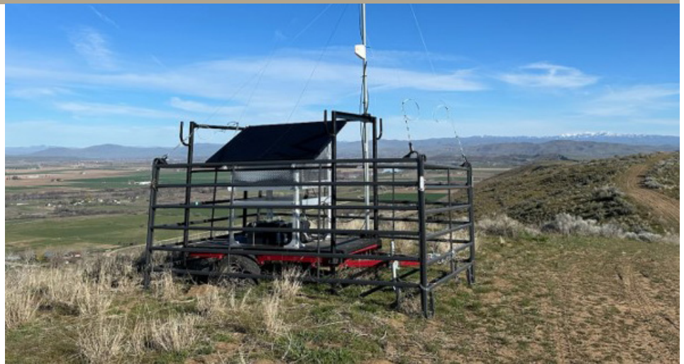
Virtual Fence base station purchased and built by the Payette National Forest and the OX Ranch for the grazing pilot project. Here the base station is set up above the training pasture near Payette, Idaho. (Courtesy Payette N.F.)
