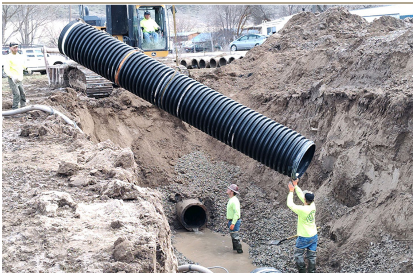
Contractors position new drain pipe into position for the Payette SWCD and Canyon County Drainage District #2. The project has been completed in time for the 2025 irrigation season. (Photo by Meghan Brooksher/SWC)
