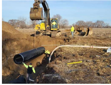
WQPA Underground Drain Replacement Phase II In FY2025 Phase II replaced a further 160' section of failing concrete pipe.
