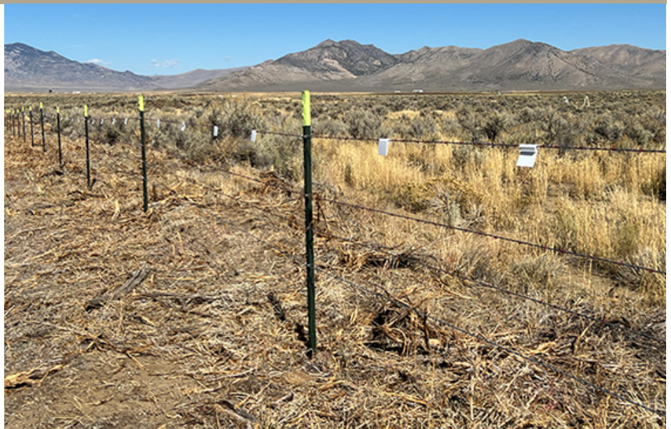
Wildlife-friendly fencing includes special reflective markers on the top strand that alert sage grouse and big game animals that they're approaching a fence in the daytime and at night. (Photo courtesy of IDFG).
