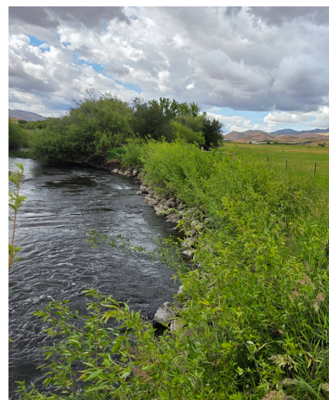
Contractor works on the Spiker streambank-stabilization project, which treated 460 feet of the streambank. Below right, the Spiker project a year later, showing the willows flourishing. (Photos by Meghan Brooksher, SWCC)
