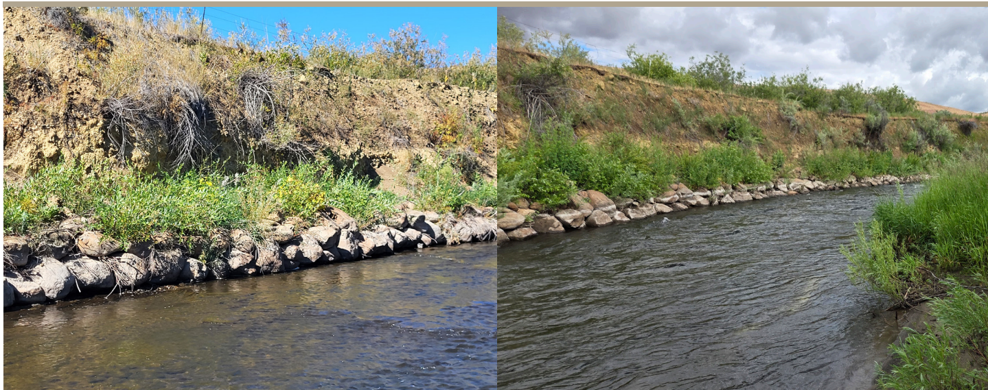
Left, rock riprap and willows are in place for the Younie Ditch streambank stabilization project. Right, another view of the stabilized streambank, looking upstream. (Photos by Meghan Brooksher/SWCC)
