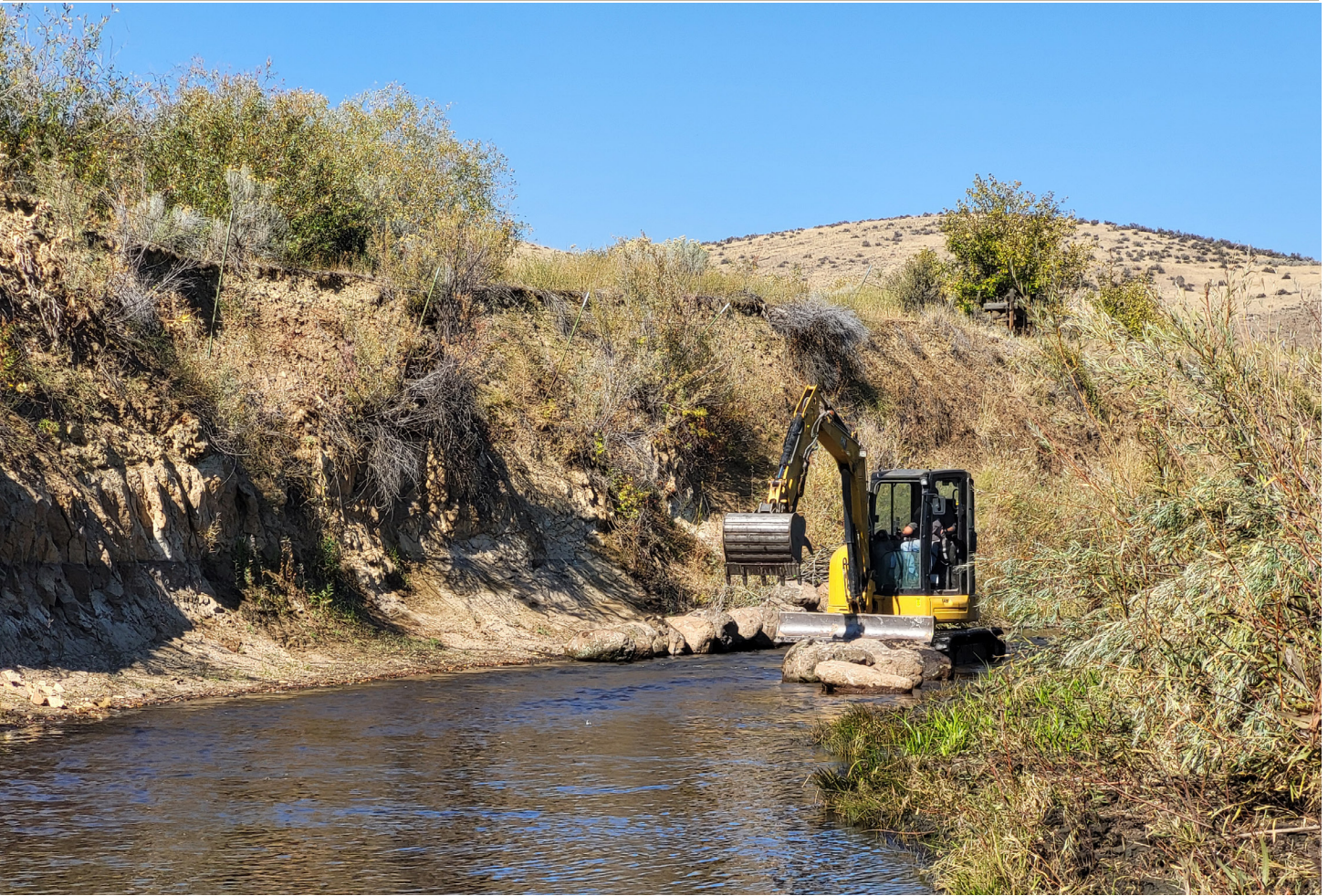
Contractor begins placing heavy rock at the base of an eroded streambank on Squaw Creek, near Ola. The project was badly needed because the bank erosion threatened the integrity of the Younie irrigation ditch. (Meghan Brooksher photo)
