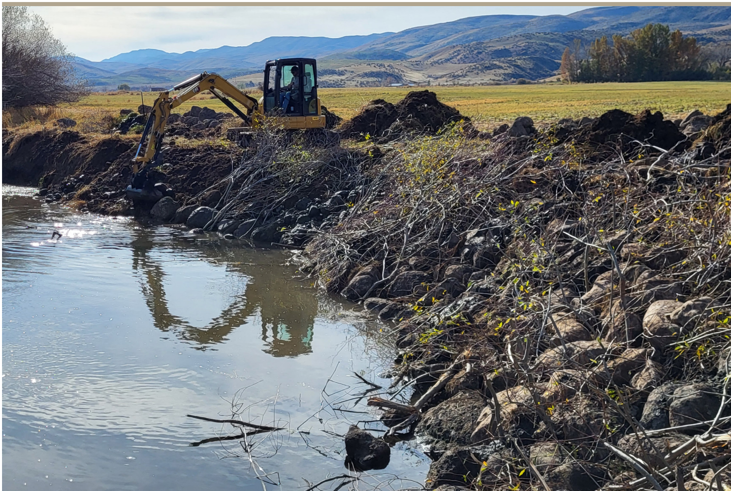
Contractor works on the Spiker streambank-stabilization project, which treated 460 feet of the streambank. Below right, the Spiker project a year later, showing the willows flourishing. (Photos by Meghan Brooksher, SWCC)
